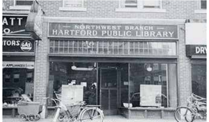
Northwest Branch in 1940 at 1239 Albany Ave.
